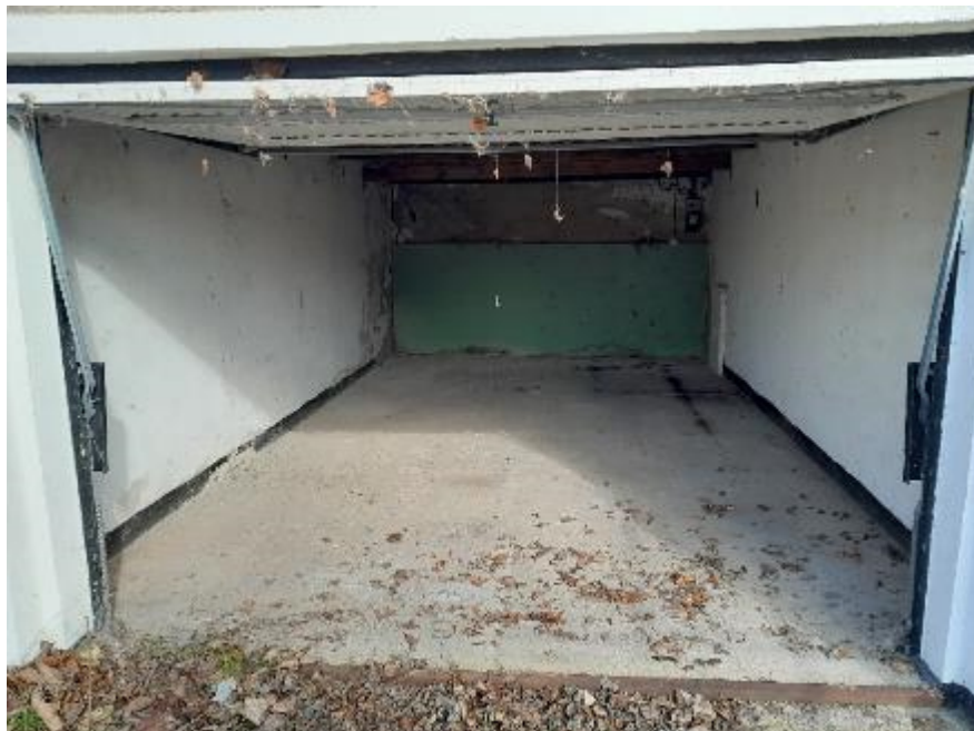
Foto 9: Blick in Garage 2
