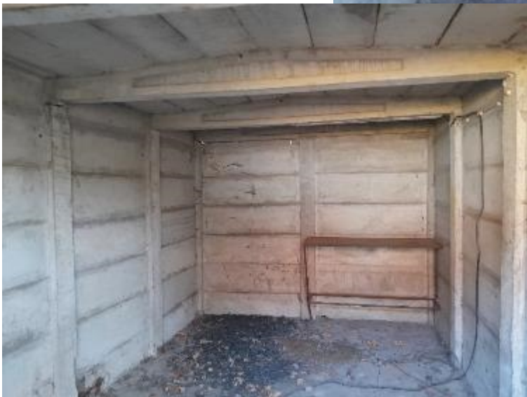
Foto 45: Blick in Garage 3
